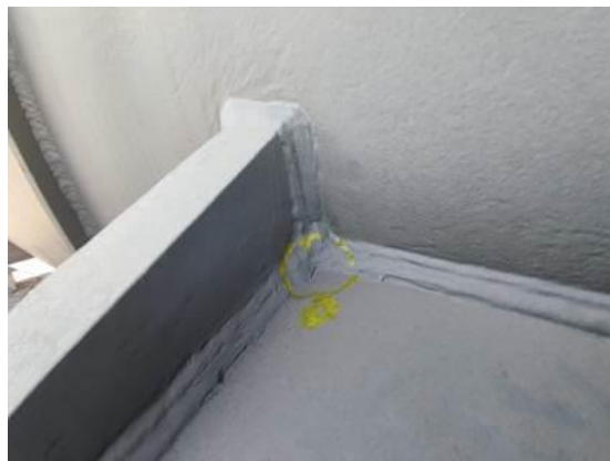
Gambar 9. Defect Cracking
