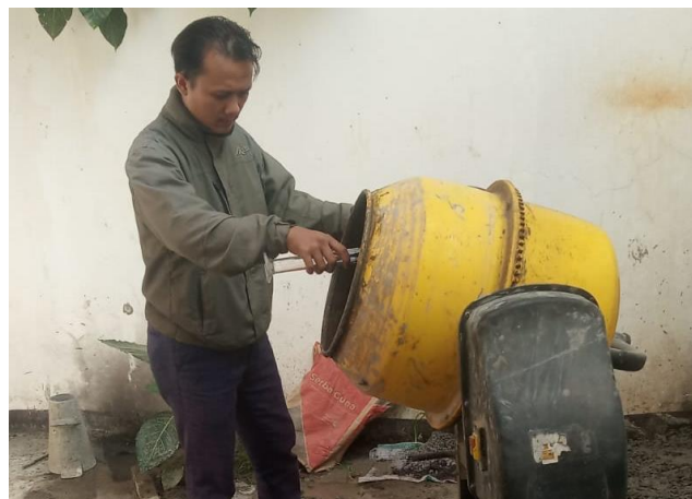
Gambar 2. Penambahan Gula Pasir Kedalam Campuran Beton
